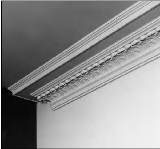
Installation of cornice - 6313
