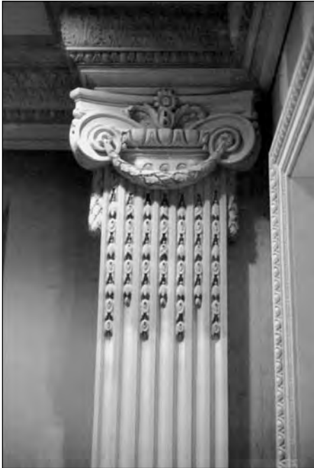
Pilaster Capital installation
